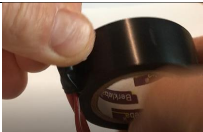
4. Apply 2 half lapped layers of vinyl electric tape for mechanical protection
