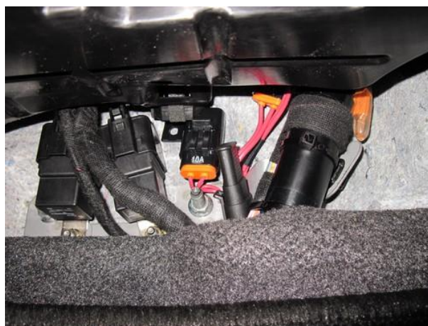
Fuses when finished.
