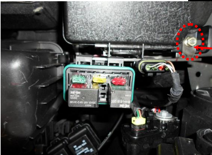
Fuse relay box and diagnose connector .
