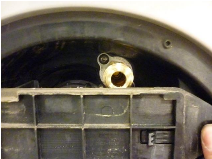
Glue on the 50mm extension pipe
